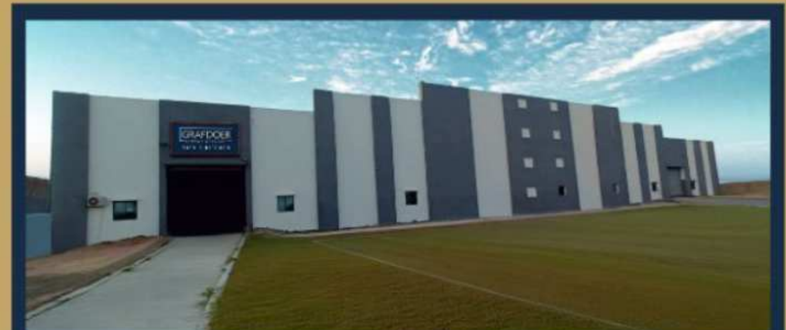
Sanitaryware Plant at Morbi
